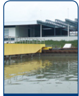
Wastewater Treatment Plant, Lyon, France, Large Diameter
