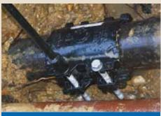
During bolt up repair clamps deform to take the shape of the pipe
