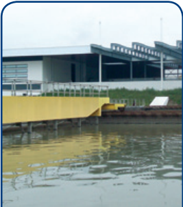
Wastewater Treatment Plant, Lyon, France, Large Diameter
