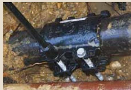
During bolt up repair clamps deform to take the shape of the pipe
