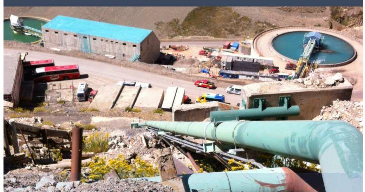
Project Sector: Mining Client: Tubexa / Coddler **Distributor: Felmat Chile** Specification: Large Diameter Stepped Couplings (DN1000) Year: 2014
