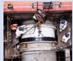
New bespoke Large Diameter Flange Adaptor being installed
