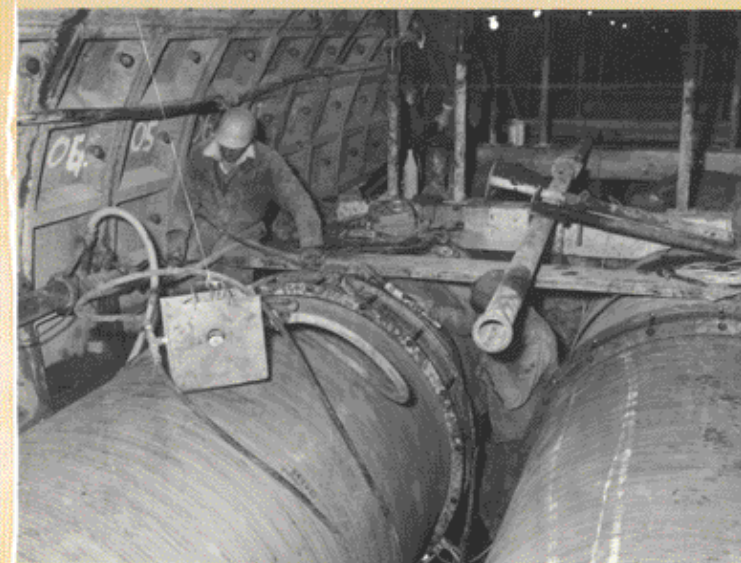
Tyneside Interceptor Sewer June 1975. 55 1/2" V.I.C. on Redlands GRP pipe.
